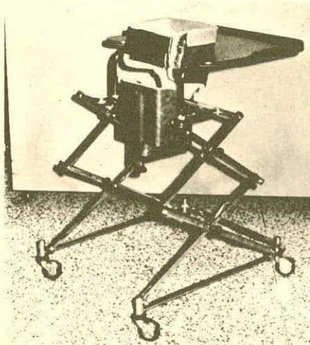
Figure 5: Adjustable pommel walker modified for increased trunk support.
