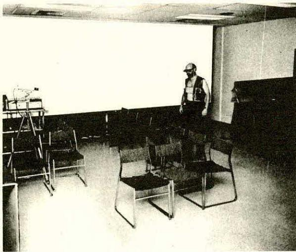
Fig. 4. Sensory aid as worn in mobility course. Suspended overhang (right), chairs and table with videotape recorder and TV camera (left) for recording performance of subjects.
